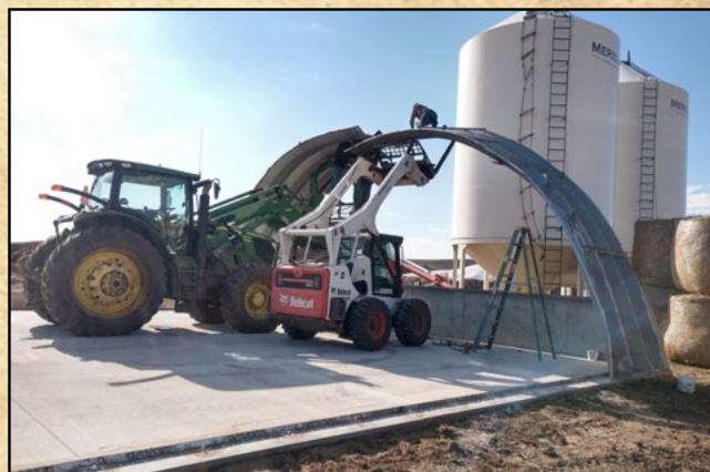
John Ross and South African employees reassembling a quonset this past fall.
